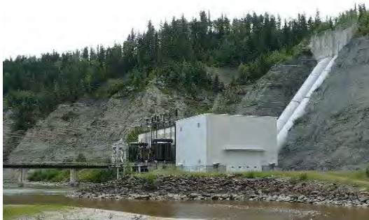
Brazeau River Power Plant
