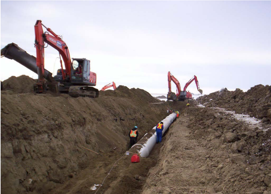
Figure 10. Installing a pipe to reduce seepage and evaporation
